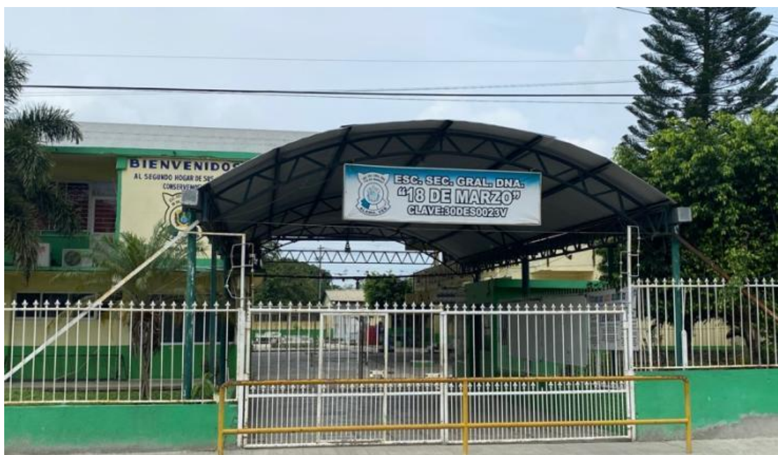
Figure 7: 18 de Marzo secondary school facade
