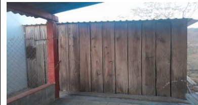
Bodega de Material Material Primaria Federal
